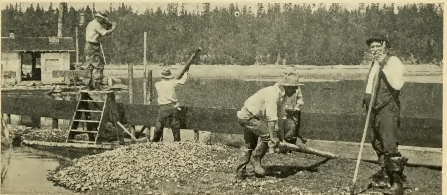
Building creosote lumber dikes by Olympia Oyster Co. J. Y. Waldrip, foreman, on right.
